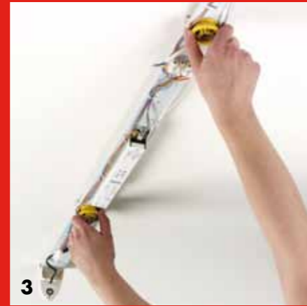
3 Offer up the spine plate (see below) and, using the yellow snap ratchets, push home and secure with short twist (see above)
