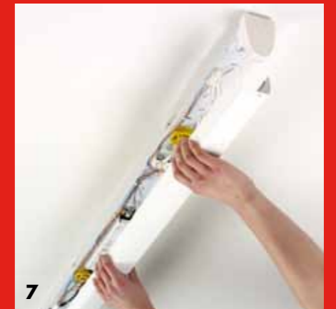
7 'U' shaped cover 'snaps' onto the spine plate
