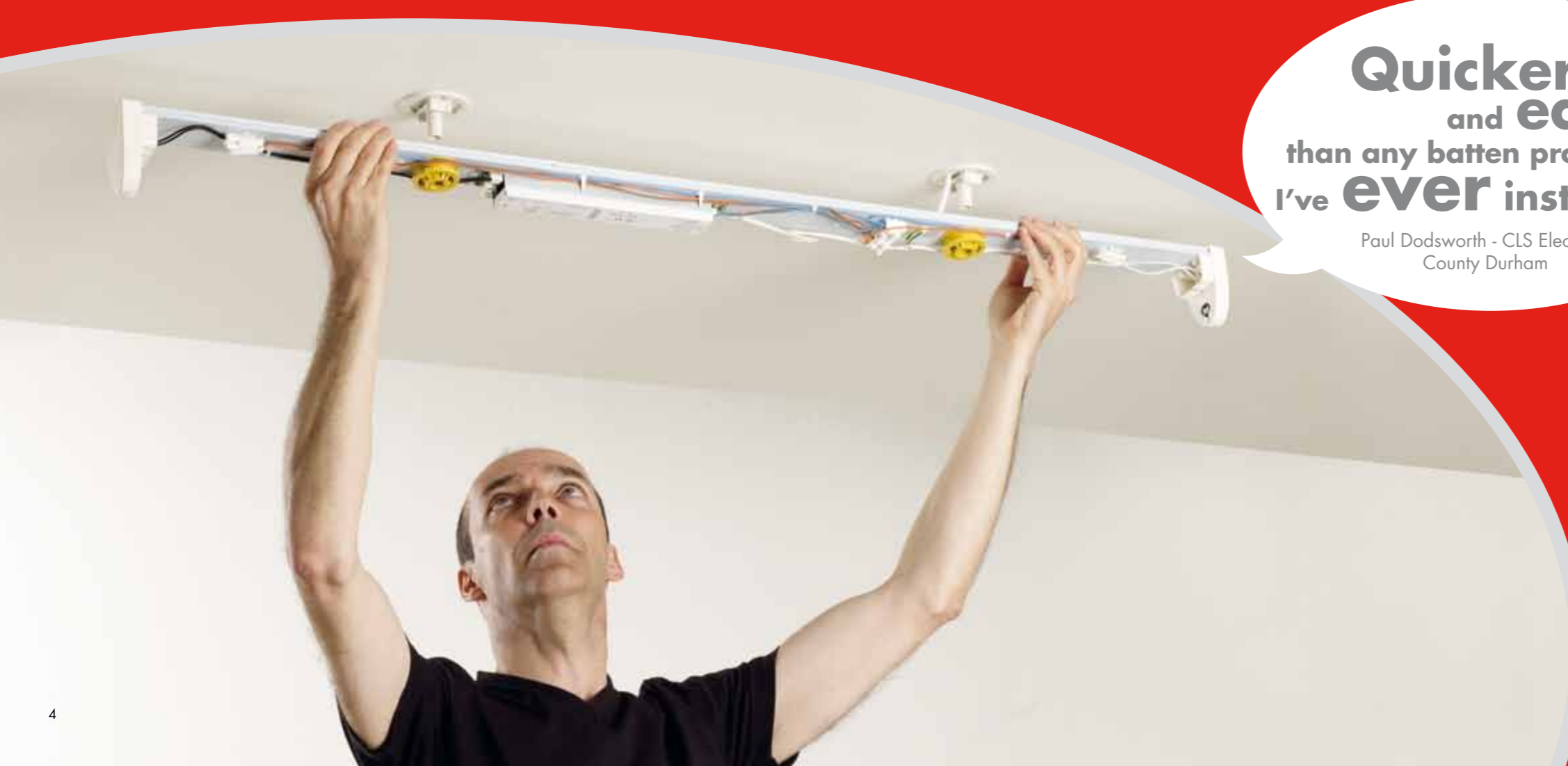
3 Offer up the spine plate (see below) and, using the yellow snap ratchets, push home and secure with short twist (see above)
