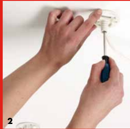
2 Fix mounting plates to the surface/BESA box, using the fixing centres template if required
