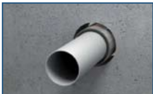
4. Slide the sleeve into the aperture and centre it
