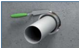
5. Fill the opening with acrylic, foam or mortar
